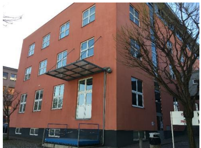
Building D – Rear Façade
