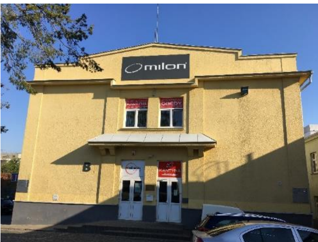
Building B - Exterior
