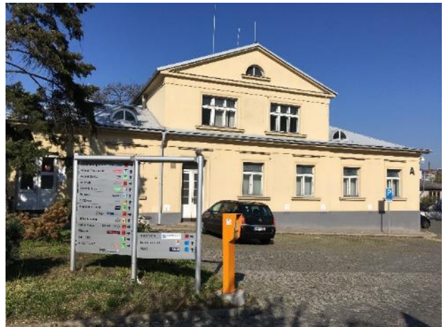
Building A – Exterior
