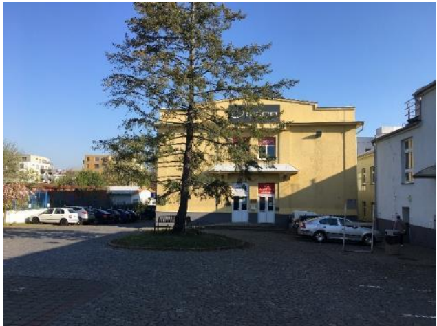
Office Park Hlobětín Exterior
