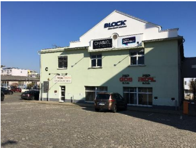
Building C - Exterior
