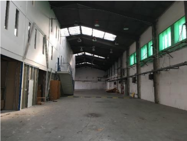
Building G – Vacant Storage
