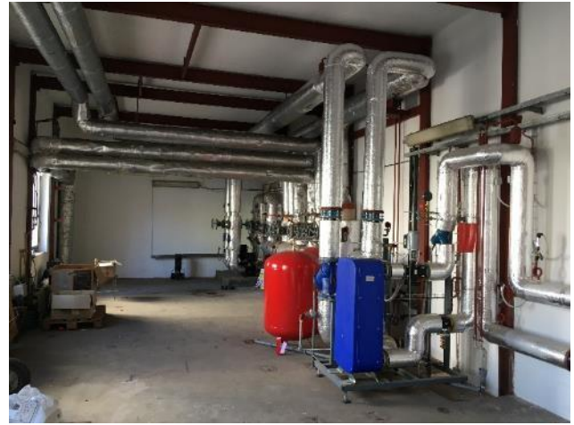
Building E – Technical Room
