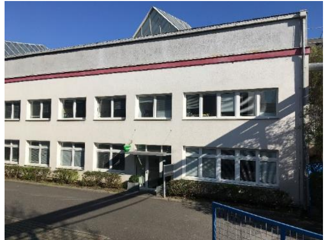
Building G – Exterior
